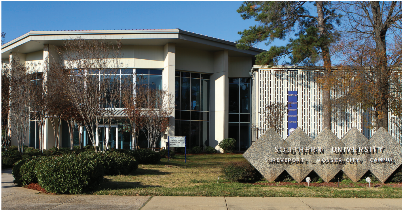
*Southern University Shreveport - Admin Renovation
